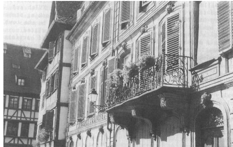
Photo 4: Place St Etienne is surrounded by various examples of Vernacular architecture well
